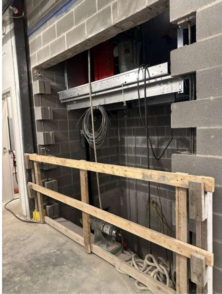
Elevator shaft CMU installation
