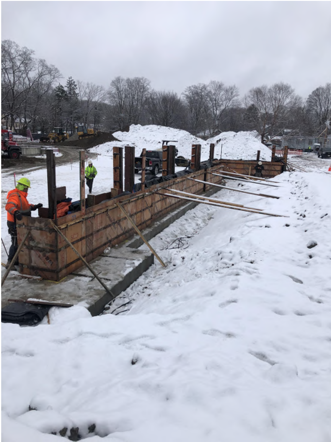
Concrete Formwork.
